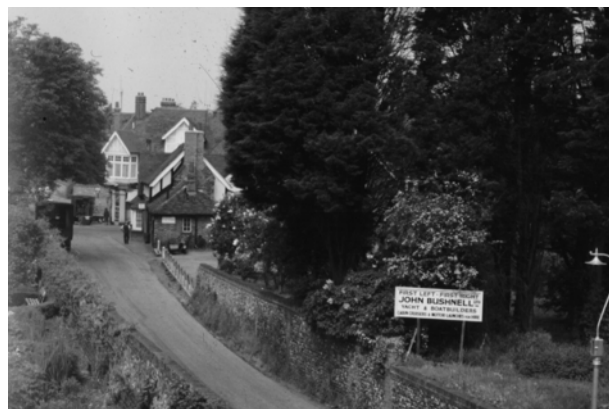
School Lane, towards the Greyhound, before the car park was built
