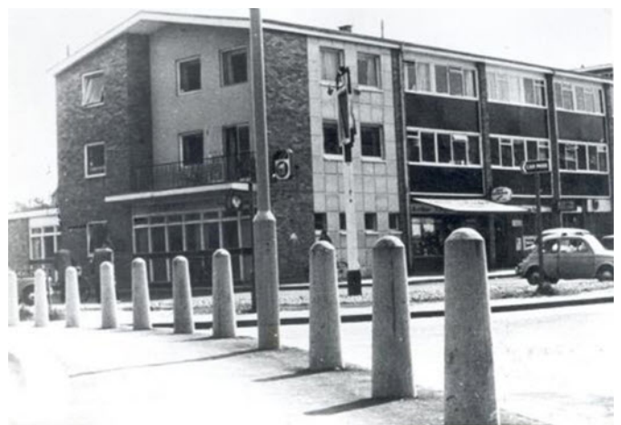
Crockhamwell Road shopping precinct, with the modern Chequers pub on the left
