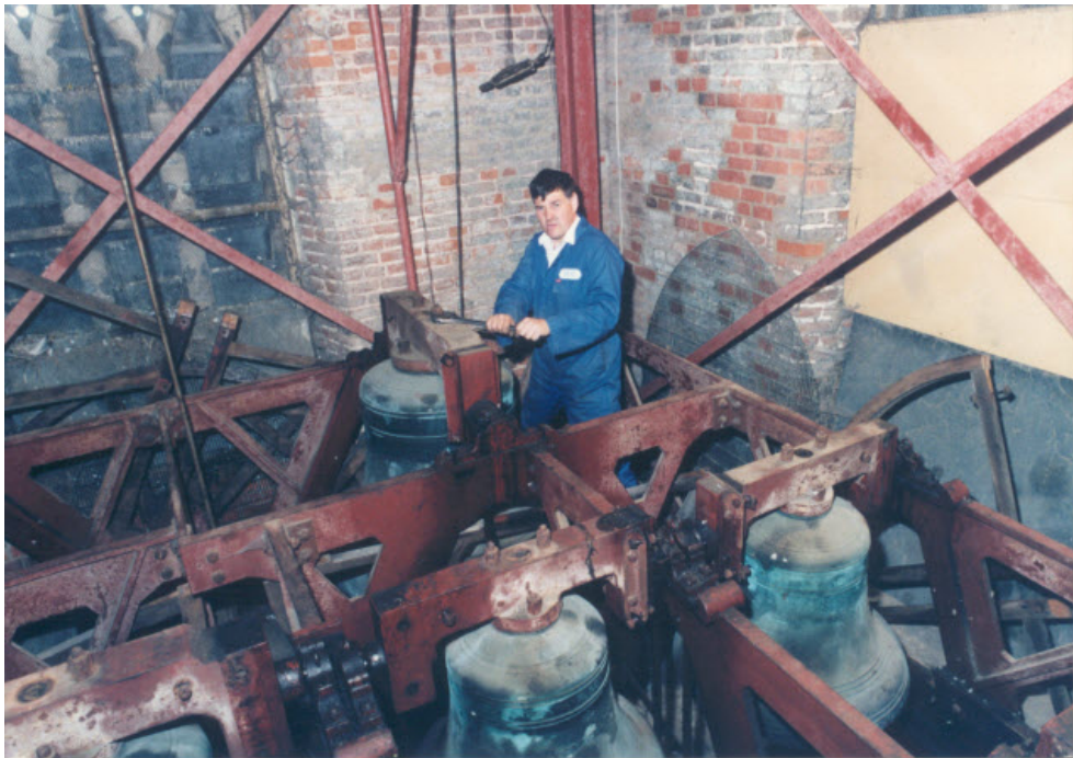
Three of the bells in the "down" position, under maintenance.
